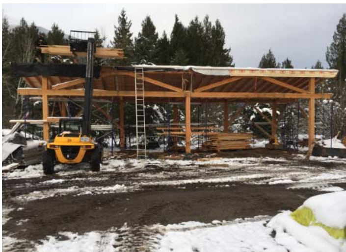
New lumber storage shed
