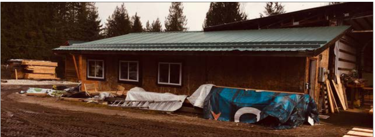
The old kiln is being retrofitted as a staff break room
