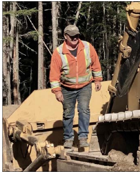
Ray Dosenberger building road in West Harrop
