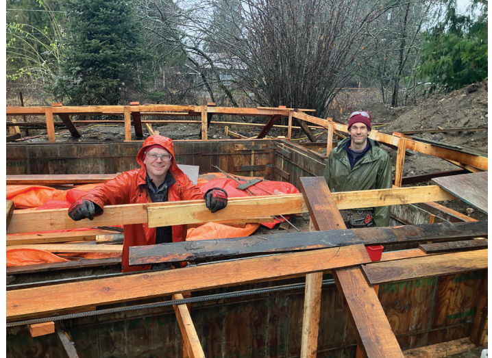
Carpenters Jacques and Raphael working on the moulder building extension
